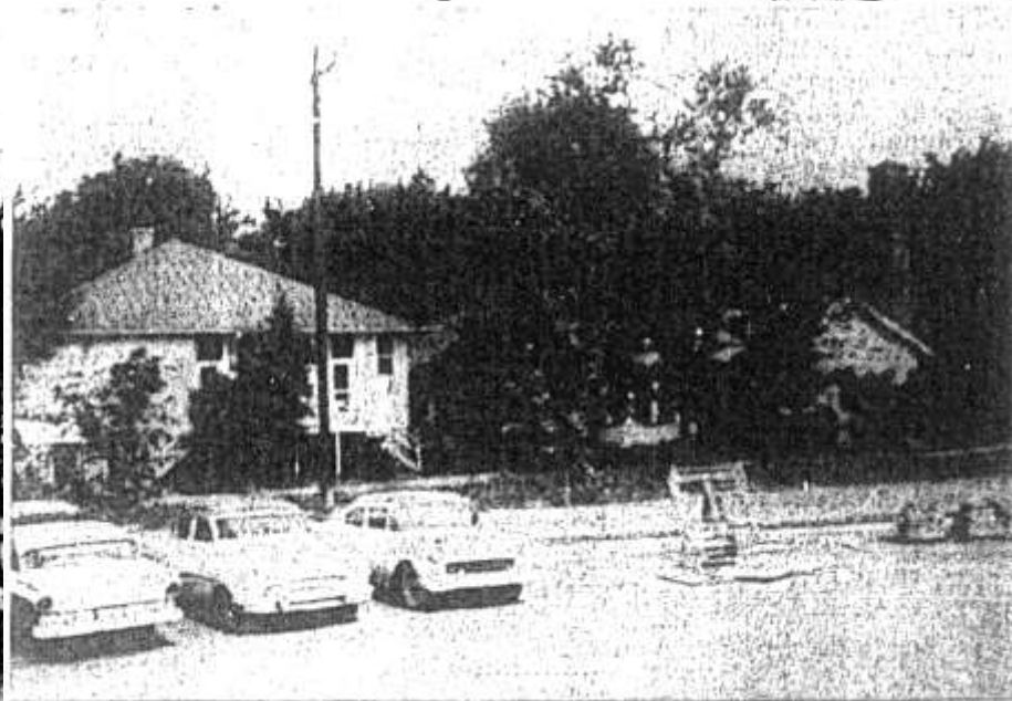
Foliage and trees obscure this shot of the old Greathouse School, taken from the Sears Rnebuok property next door.
